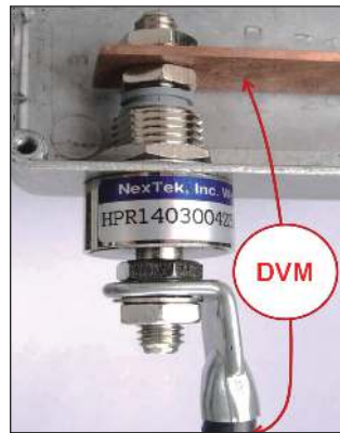
Fig. 4. Measuring Total Voltage Drop
